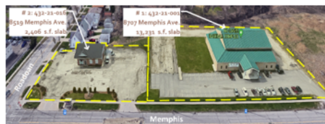
Remove and Properly Dispose Potentially Hazardous Materials at:
